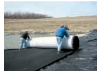
The first step is to roll Zeomat out across top of lagoon.
