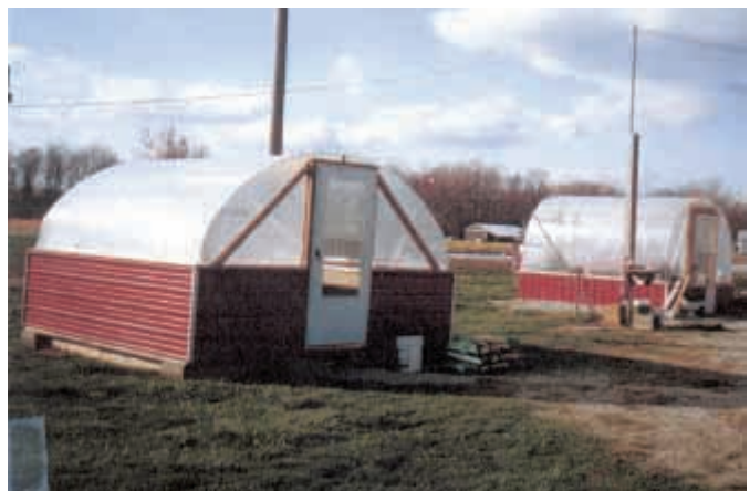
Joe Leihgeber builds greenhouses on skids so he can move them wherever he wants.
