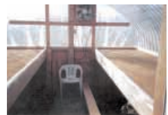
Cattle panels form the frame of 8-ft. high greenhouses which have tables, a fan, electric heater and shutters.
