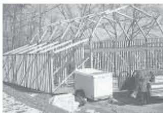
Elimination of trusses provides a building with more usable space (left). Design eliminates need for load-bearing headers for trusses to sit on.
