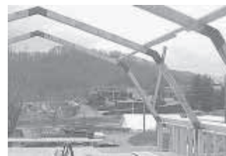
Elimination of trusses provides a building with more usable space (left). Design eliminates need for load-bearing headers for trusses to sit on.
