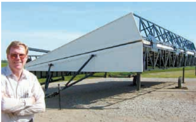
The 33 by 50-ft. building folds in half lengthwise to 16 1/2 by 50 ft., making it narrow enough to be pulled behind a 1/2-ton pickup down rural roads and over bridges.
