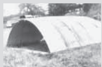
Grain bin panels were used to put together this goat shelter (left). Panels are bolted to a wood framework that mounts on skids, making shelter easy to move.
