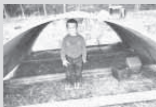
Grain bin panels were used to put together this goat shelter (left). Panels are bolted to a wood framework that mounts on skids, making shelter easy to move.
