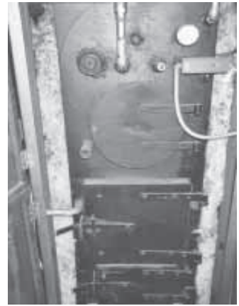
Ziegler started with a 1947 Heil gas boiler and built a new housing around it (left). Corn is augered out of a metal hopper alongside boiler.
