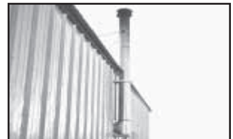
He uses 5-gal. buckets to dump corn into hopper (left). A 6-in. stainless steel stack vents exhaust out of boiler.
