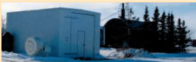
Wilfred Mollenbeck and his two sons built this big bale furnace from a giant 13,000-gal. fuel tank measuring 21 ft. long and 13 ft. in diameter, right. Heated-up water from furnace goes to heat exchanger in building on left.
