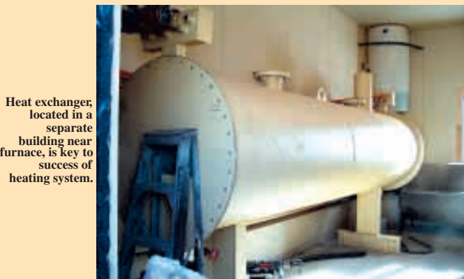
They cut a hole in one end of tank and inserted a 19-ft. long by 7-ft. dia. rail car tank inside. After cutting the end off the 7-ft. tank, they used both tanks' end pieces to make a big double-walled door.
