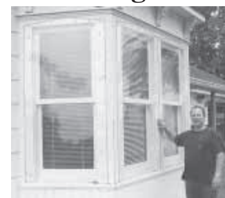
To temporarily seal up windows on an old house he moved into, George Marley screwed sheets of clear plexiglass to the outside.
