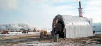
Insulated sheet metal housing was built around furnace. Note chimney on back end.
