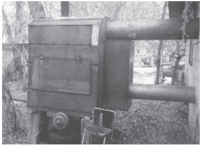
Outdoor "hot air" wood furnace was built out of an old wood stove. Sheet metal housing around stove is fitted with a squirrel cage fan that blows hot air through two big pipes running to house.
