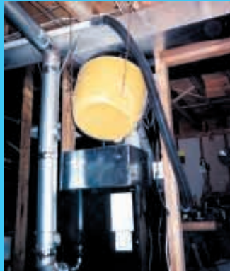
Corn moves about 30 ft. from outside bin to shop vac, which hangs above corn furnace. Corn simply drops out of shop vac into furnace hopper.
