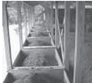
Eleven compost bins run down one side of building.
