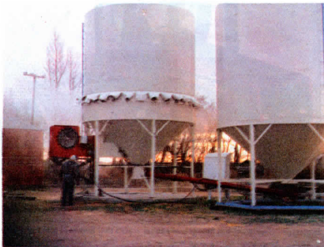
Loyns modified a conventional 2,000-bu. bin to make recirculating batch dryer.
