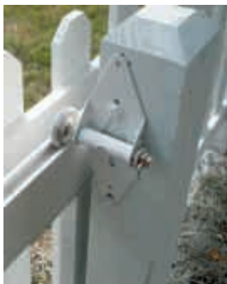
Rollers are on adjustable plates so they can be moved up or down to adjust gate height.
