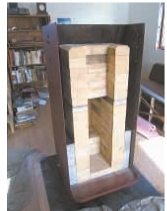
Efficient wood stove is basically a small masonry heater with a steel skin. Firebrick stores fire's heat and also allows you to make a hotter fire.
