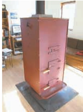
Efficient wood stove is basically a small masonry heater with a steel skin. Firebrick stores fire's heat and also allows you to make a hotter fire.
