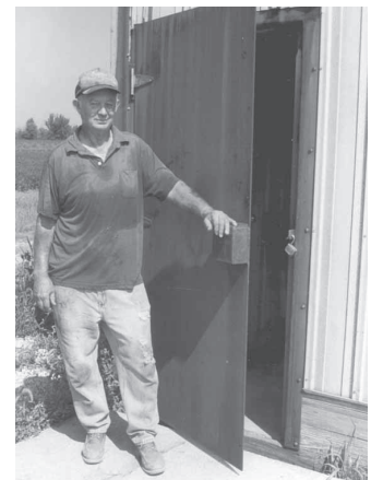
To keep thieves away, Gale Courson made this steel plate outer door equipped with a deadbolt and hooded padlock shield.
