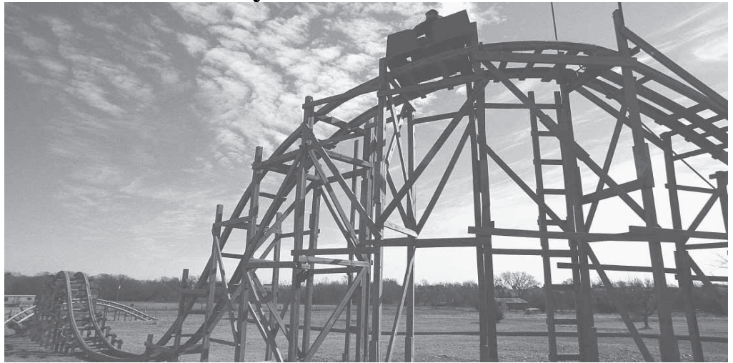
Jeremy Reid, an engineer, wrote several computer programs to calculate data for the track profile and to demonstrate the aerodynamics of his design for the roller coaster he built in three years. Lumber, screws, nails and other parts cost about $5,500.
