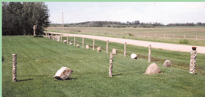
Tired of people driving on his lawn, Laurent Terrault decided to build a rock fence. Sucker rod and stucco wire is used to hold the rocks in place.
