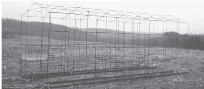
"My husband had extra rebar around, so we welded it together to form a framework to hold cages and to support the tarp for an exterior," says Tammy Miller.
