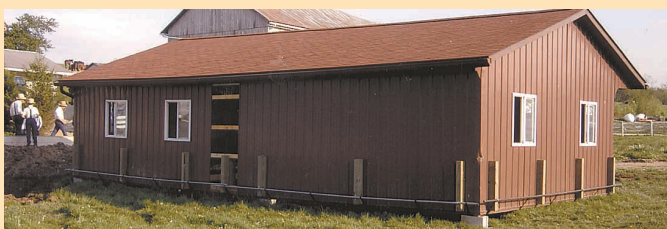
Dennis Miller moved this 24 by 50-ft. storage building about 100 ft. with the help of a few neighbors. Prep work involved attaching a 1 1/2-in. pipe to the perimeter of the building.
