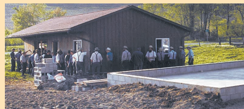
Dennis Miller moved this 24 by 50-ft. storage building about 100 ft. with the help of a few neighbors. Prep work involved attaching a 1 1/2-in. pipe to the perimeter of the building.
