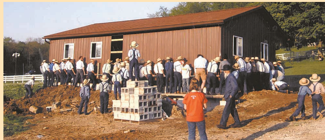
Dennis Miller moved this 24 by 50-ft. storage building about 100 ft. with the help of a few neighbors. Prep work involved attaching a 1 1/2-in. pipe to the perimeter of the building.
