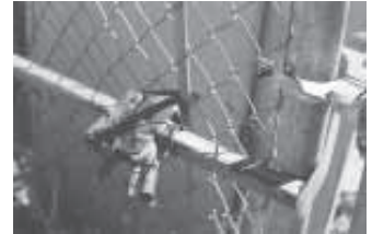
To use, simply hook the jack's small carriage hook into the fence and put the top around the post. Then crank the jack to tighten.
