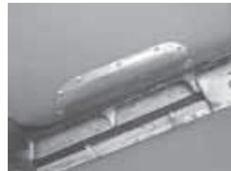
Strips attach into poly with self-tapping screws.
