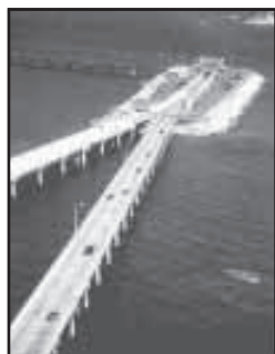
Photo shows one point where the Chesapeake Bay Bridge heads underwater to allow ships to pass.
