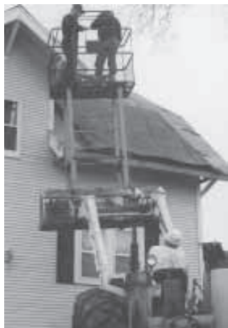
Scaffold stands about 8 ft. above the loader bucket, which means a person standing in it can reach up to about 27 ft.
