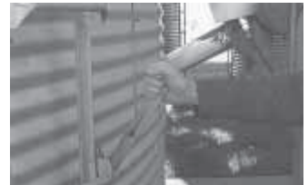
Cable runs down side of bin to lever, which is used to pull catch pan out of way when grain is being loaded into bin.
