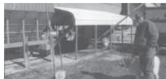
The Elliot brothers use a fiberglass carport to protect grain drying components.
