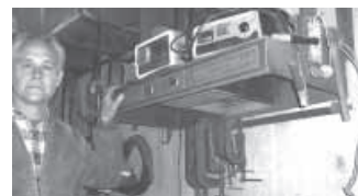
Bob Bugger bolted this old oven range hood to the wall of his basement to pull fumes out of his house.
