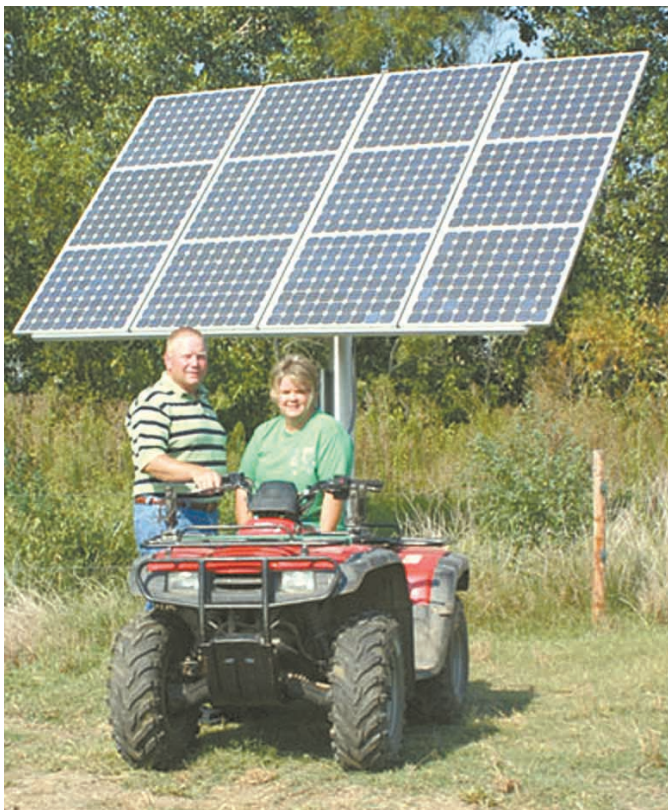
Sun Tracker solar panel is used to pump 10,000 gal. of water a day to Fricke's cattle.
