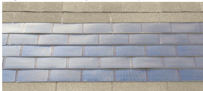
Shingle-type solar strips simply nail on in place of asphalt shingles.
