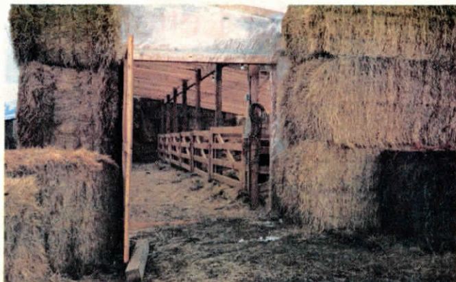
The 70 by 32-ft. shed features a clear plastic roof and straw-bale sidewalls.
