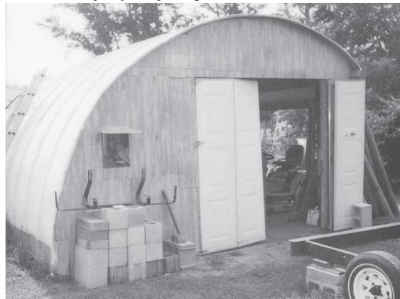
Roy Gray built this low-cost shop by laying panels from an 18-ft. dia. grain bin over on their side.
