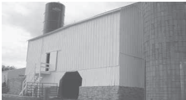
Barn restored to its former glory.
