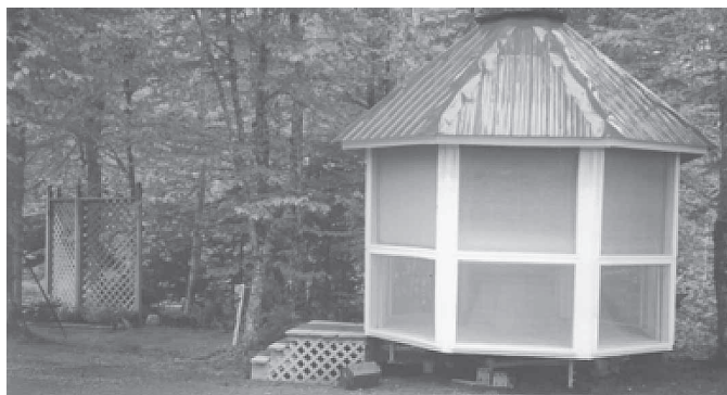
Walter Rodler can tow this gazebo to different spots in his farm yard. It rotates on a 10-ton semi tractor axle.
