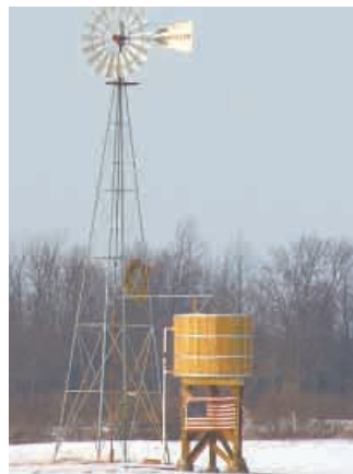
Tower's legs were made from 6 by 6-in. treated lumber with 2 by 10-in. planks for cross-ties.
