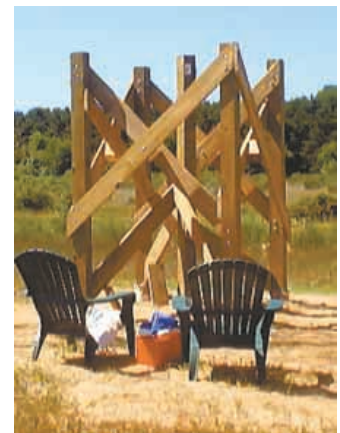
Tower's legs were made from 6 by 6-in. treated lumber with 2 by 10-in. planks for cross-ties.
