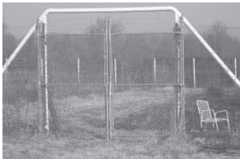
Nachamkin used 3-in. dia. pvc pipe to make an 8-ft. deer fence around his half-acre garden.
