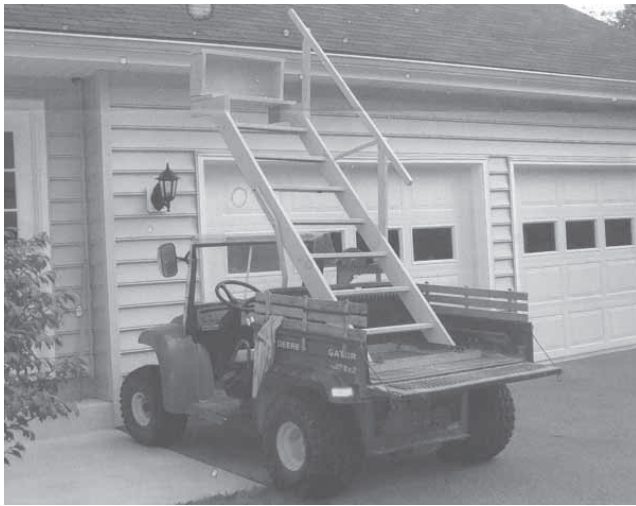
"It's very stable and isn't top heavy at all. In fact, it's much more stable than a ladder," says Richardson about his Gator-mounted scaffold.
