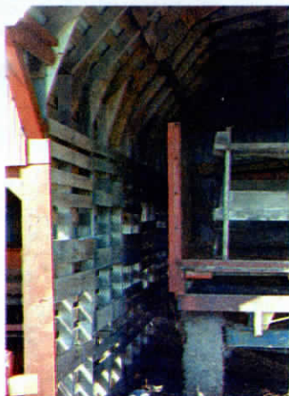
Plywood "gussets" reinforce roof sections.
