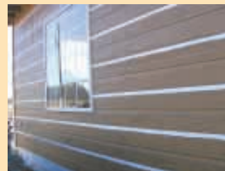
To mimic the chinking, he painted a white strip onto each siding board.
