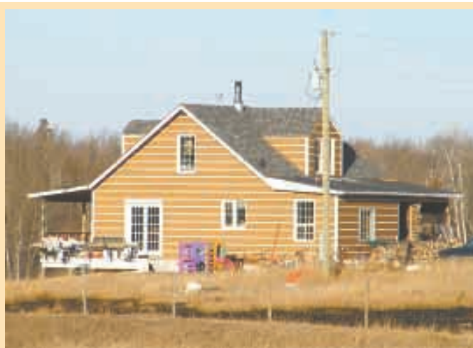
Brad Blonjeaux re-sided his house with "composition siding" because it looks like wood.
