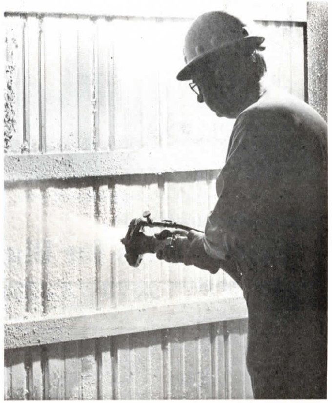
It readily adheres to metal, wood, concrete, glass or other surfaces. Can also be sprayed over foam insulation to reduce fire danger.
