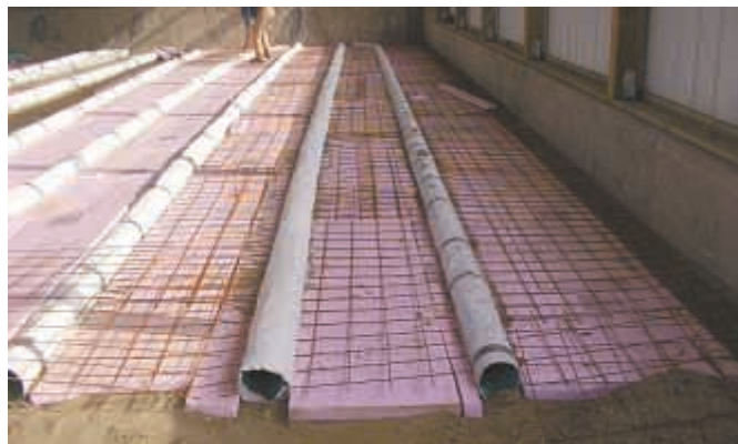
Pvc pipes are buried in the insulated concrete floor. When compost is piled on the floor the vapor inside the pipes heats up.
