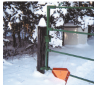
Vertical lift gate means no worrying about snow drifting against the gate.
