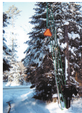
Fold-up gate's lift mechanism is an electric winch mounted at base of gate post.
