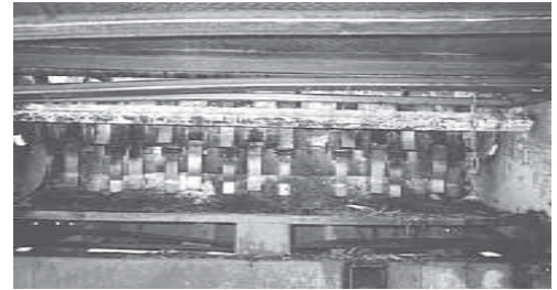
Hacault made flails out of 2 by 3/8-in. flat iron.
