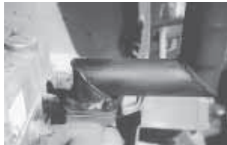
An L-shaped pipe comes off the manifold.
