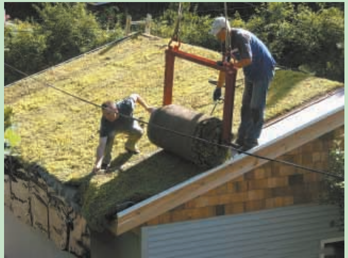
Green roofs keep buildings warmer in the winter and cooler in the summer. They should last at least three times longer and provide heating and cooling benefits.
