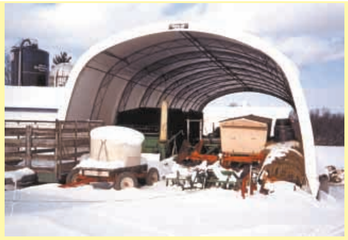
View from upper end shows equipment parked under silo roof, on top of silage.
