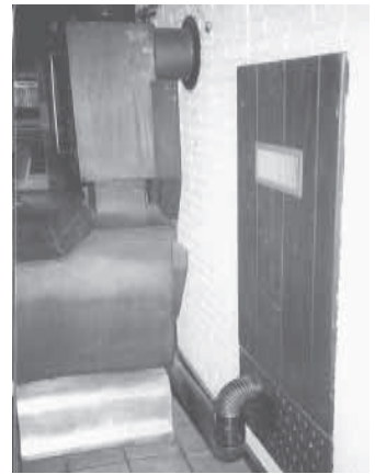
Stove has a series of open holes on front and a built-in “recovery unit” on top (left). Evenly-spaced tubes run horizontally through recovery unit and into a manifold on back (right).
