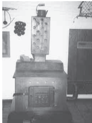
Stove has a series of open holes on front and a built-in “recovery unit” on top (left). Evenly-spaced tubes run horizontally through recovery unit and into a manifold on back (right).
