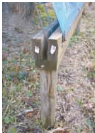
Bottom sides of arch are wedged between a pair of treated 2 by 6's that stand on top of a horizontal 2 by 4. Nails driven through the 2 by 6's hold panel wire in place.
