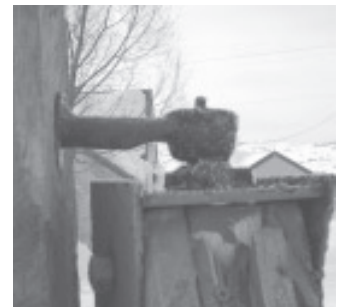
Gate hinge makes use of tie rods salvaged from old cars or trucks.
