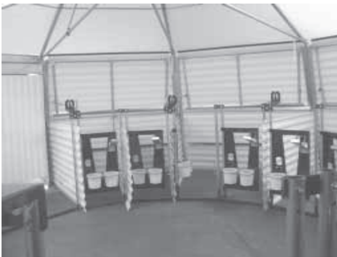
The 24-ft. dia. model has 11 pens. A larger 30-ft. model has 19 pens. Space is left at the center for a feeding and working area.
