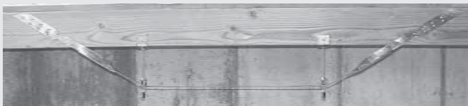
Joist Jack is a 6 1/2-ft. long steel strap that adds strength to the center of a truss across a 7 1/2-ft. span.
