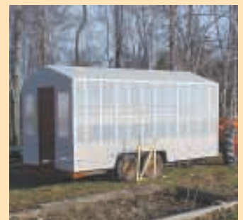
He cut a hole for a fan at one end and a doorway at the other end.
