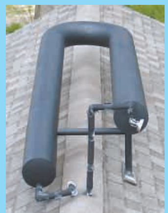
Larry Brewer's solar water heater consists of a 24-ft., U-shaped pipe painted black and mounted to the ridge of his roof. It reduces his energy costs for six months of the year.
