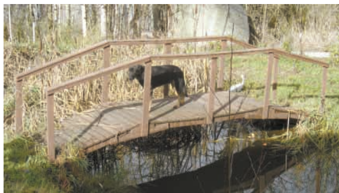
Bridge measures 18 ft. long and is made entirely from roughsawn Douglas fir.
